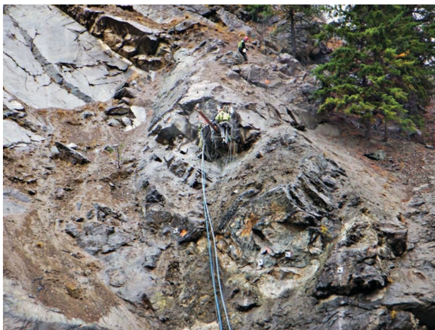
Figure 3: Drilling operations on a steep slope.
