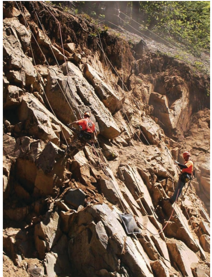
Figure 4: Scalers working off of a two-rope system.
