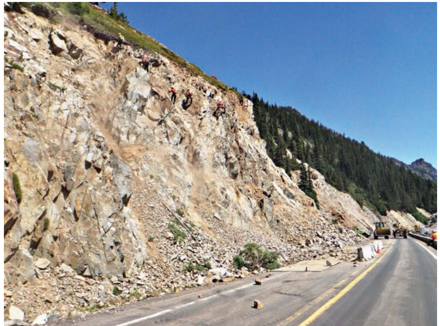
Figure 1: Scaling operations along Highway SR 410 in Washington.
